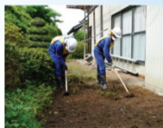
Yard: Removal of topsoil
