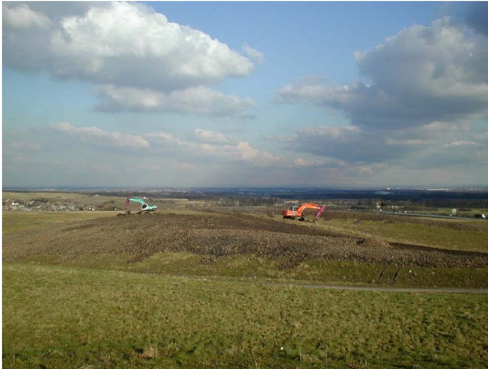
Figure 5 Decompaction of soil at Sutton Manor
