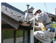
Rainwater Guttering: Removal of deposited materials
