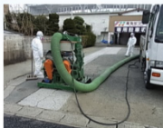
Concrete Slab: Shot blasting
