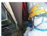
Rainwater Guttering (Downspout): High-Pressure water washing, vacuuming
