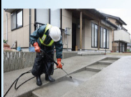
Concrete Slab: High-Pressure water washing
